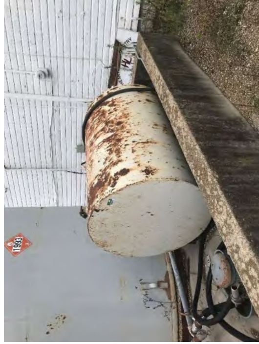
Photo #11 View of a clear diesel AST located in the AST containment area.
