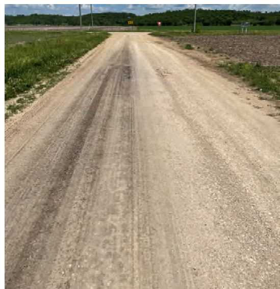
E 1300 Rd: Rutted pavement on approach N 2000 Rd
