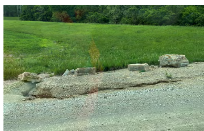
E 1300 Rd: Large rut north of N 1900 Rd
