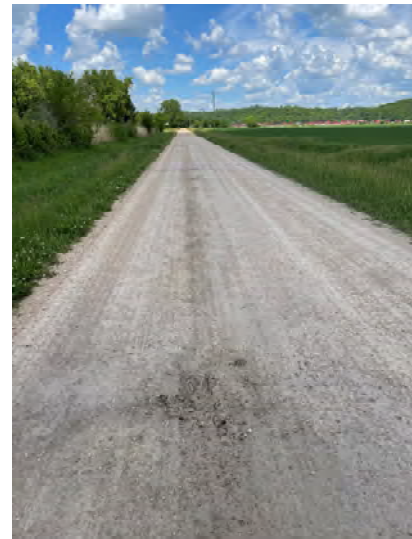
E 1250 Rd: Series of potholes north of N 2000 Rd
